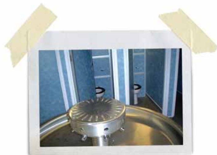
▲ Above unisex cubicles with central wash trough
